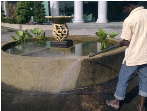
From removing fungus –
