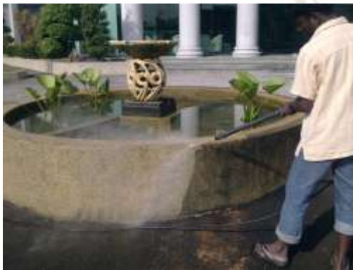
From removing fungus –
